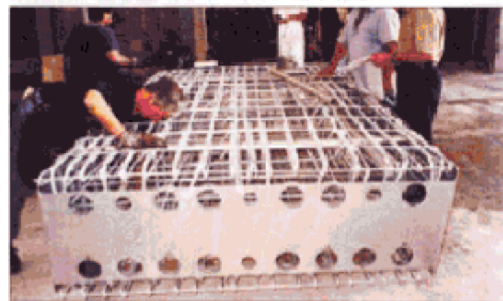
THE FINISHED CAGE IS POSITIONED IN THE FORMWORK
