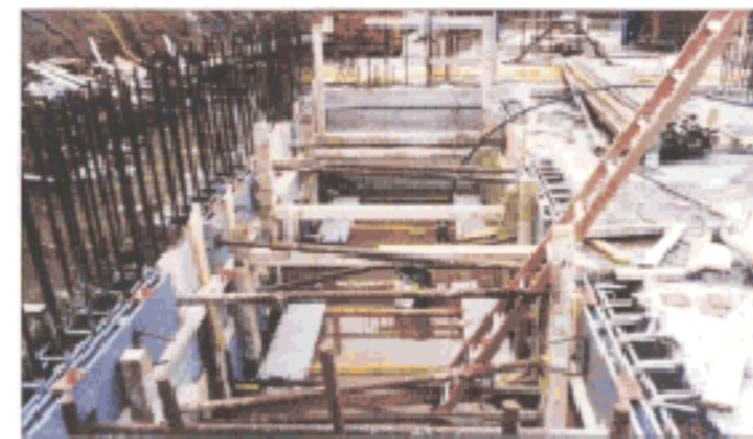
DETAIL OF THE MOLDING FOR THE SLIDING BEARING OF THE SAIL N°1
