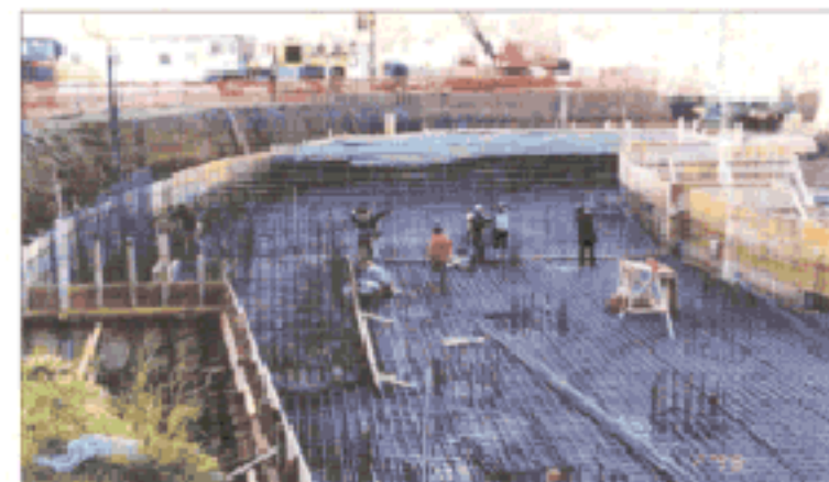
REINFORCEMENT OF THE FOUNDATION PLATE
