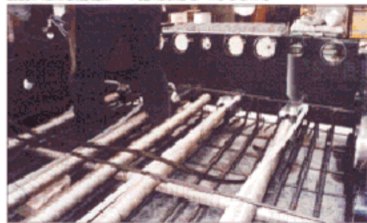
LAYING FOR THE STEEL FE B44K AND INOX REINFORCEMENT
