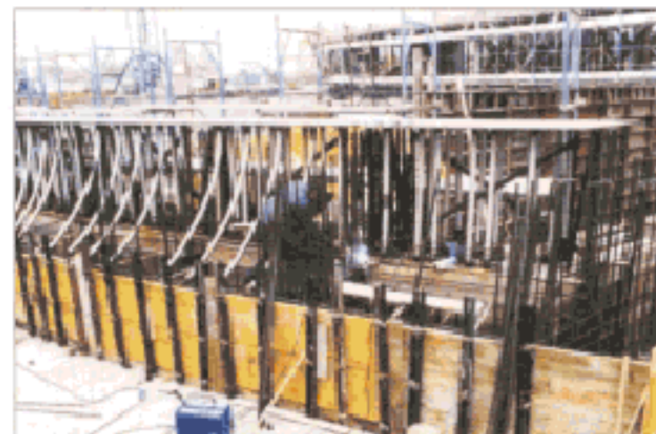
STEEL PLATES AND SHEATHS OF THE THREE SAILS
