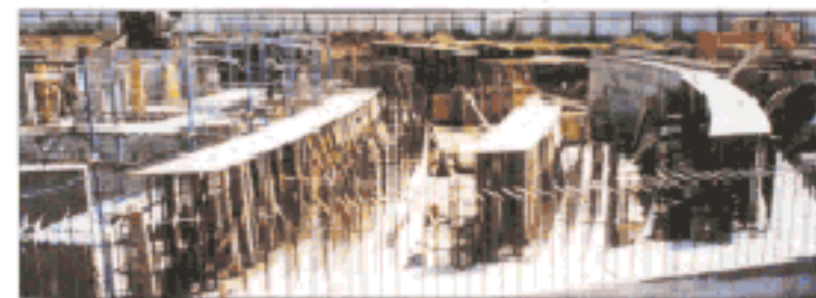
STEEL PLATES AND SHEATHS OF THE THREE SAILS
