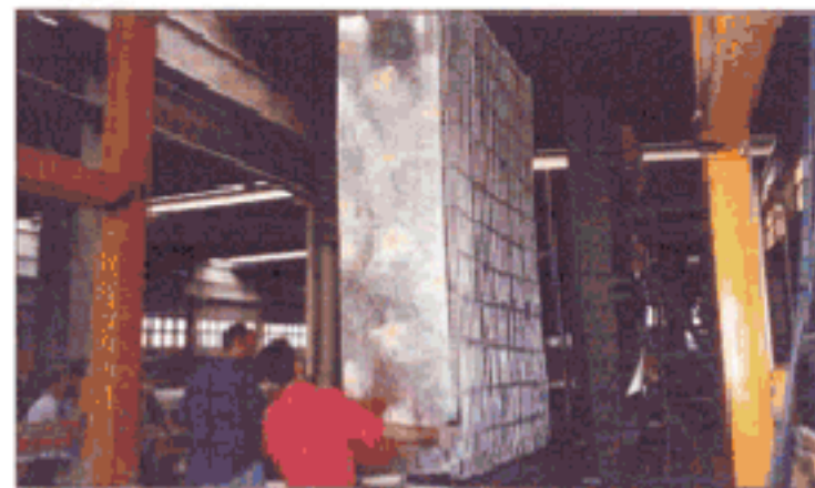
THE FINISHED CAGE IS POSITIONED IN THE FORMWORK
